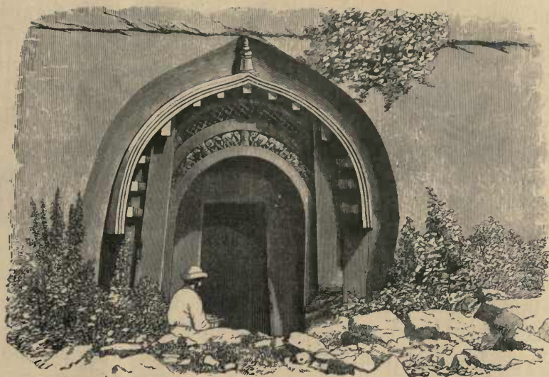
No. 3. Façade of the Lomas Rishi Cave, from a Photograph.
